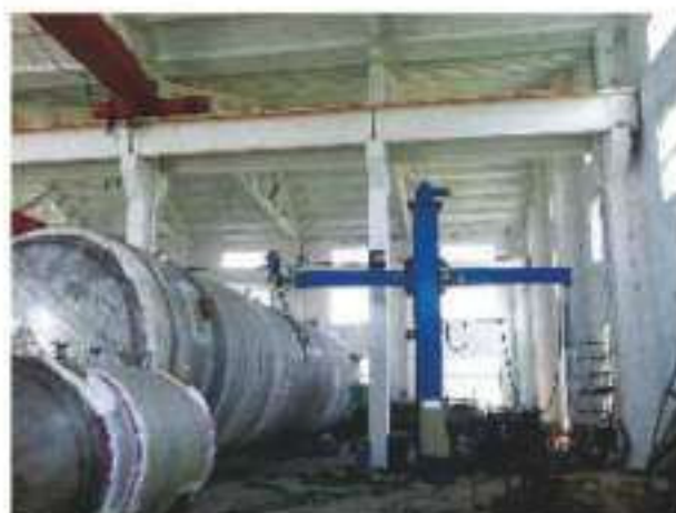
环缝焊接 Welding for circle
