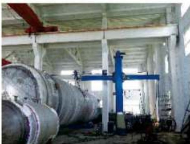
环缝焊接 Welding for circle
